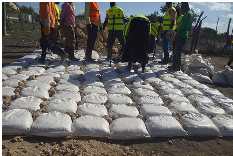
Photo 2: Do-nou's are lined up after being flattened ( http://corekenya.org/gallery/ ) to underpin an all-weather road
