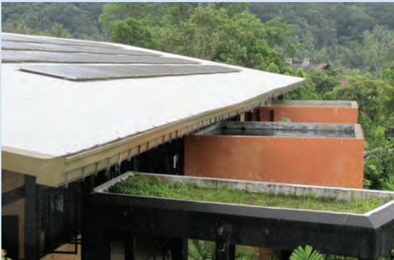
c. a Green Roof on a Model Eco-Factory
