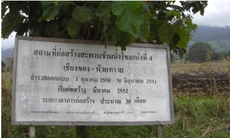
Site for the Fourth Mekong Friendship Bridge (Photograph by the author on 31 August 2008)
